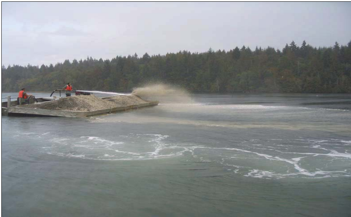
Figure 7. Graveling (frosting) over a clam bed (Corps 2015, p. 25)
